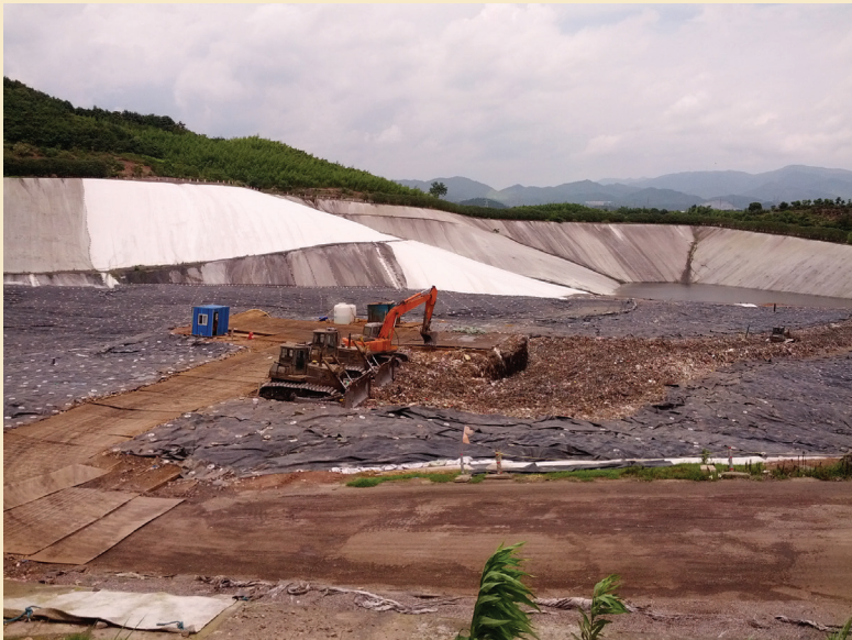
Photo 3.1 Landfill in China
